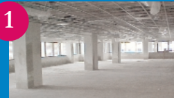
1 The ceiling grid and lighting were installed.
